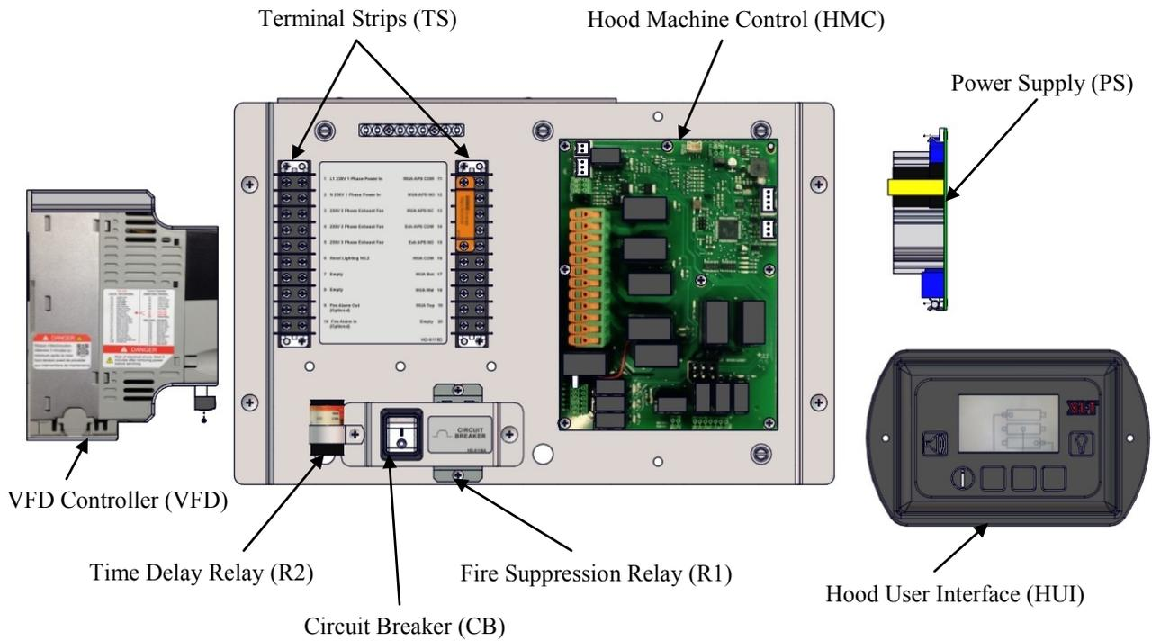
VFD Control Box (Cover removed)
